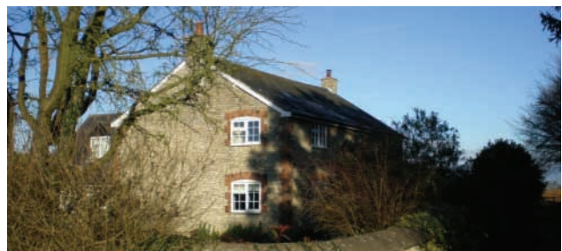
Larkwell, brick detailing in the limestone construction
